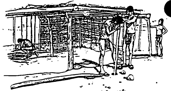
STEP 2: Building the Frame
