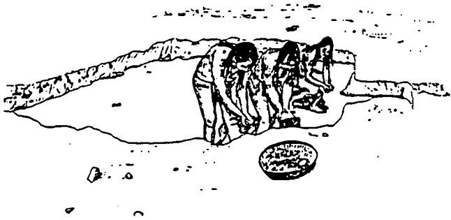
STEP 1: Plastering the Floor
